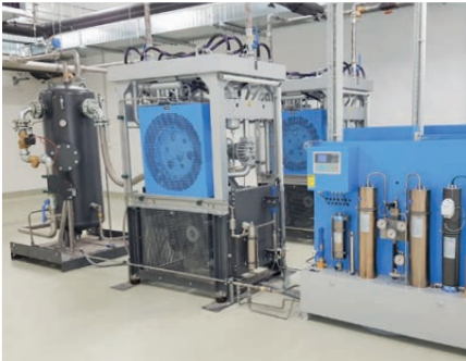
Two progressive GB 23.2 rare gas compressors operate as an interconnected unit to compress the costly helium recovered during measurement.
