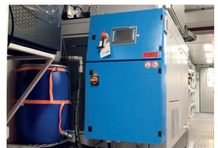
BAUER breathing-air filling system in the EIZ emergency centre.
